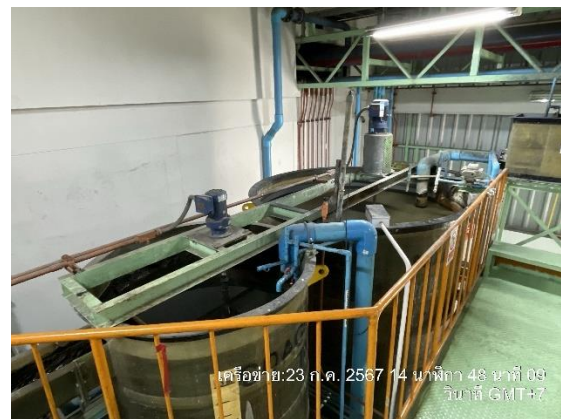
Degrease Wastewater Treatment System UT2
