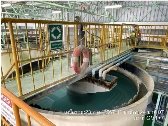
Phosphate Wastewater Treatment System UT1
